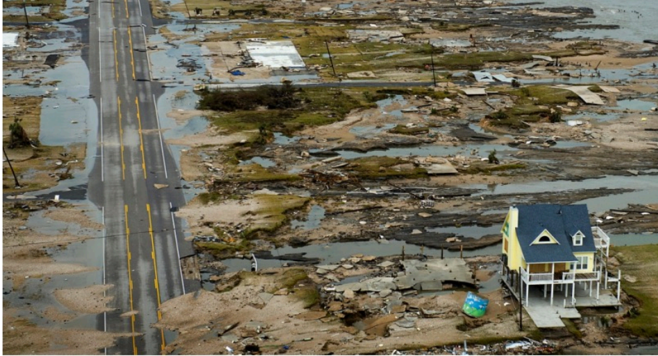
BOLIVAR PENINSULA IN TEXAS AFTER HURRICANE IKE (2008)
