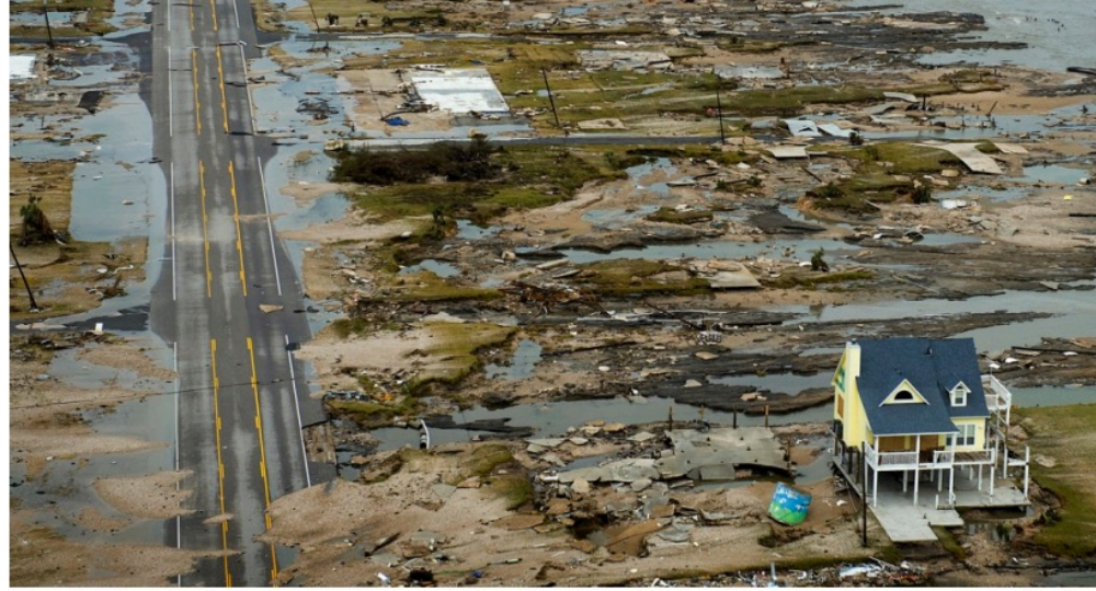
BOLIVAR PENINSULA IN TEXAS AFTER HURRICANE IKE (2008)
